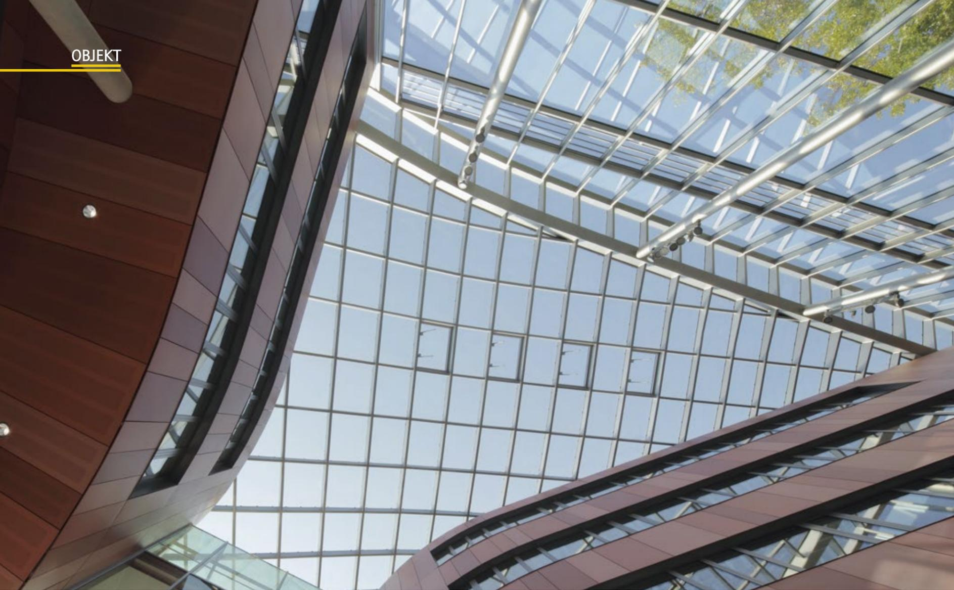
In this way, a curve was eventually reproduced with a polygon – the individual surfaces of the roof-glass-elements are flat.
