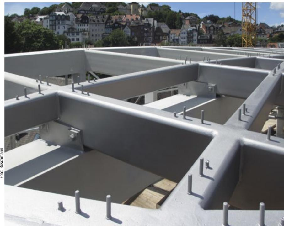
The grid of steel girders was welded on the construction site and forms an element.
