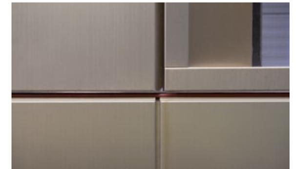
Facade detail of one of the 3.5-ton elements made of titanium-coated stainless steel sheet.
