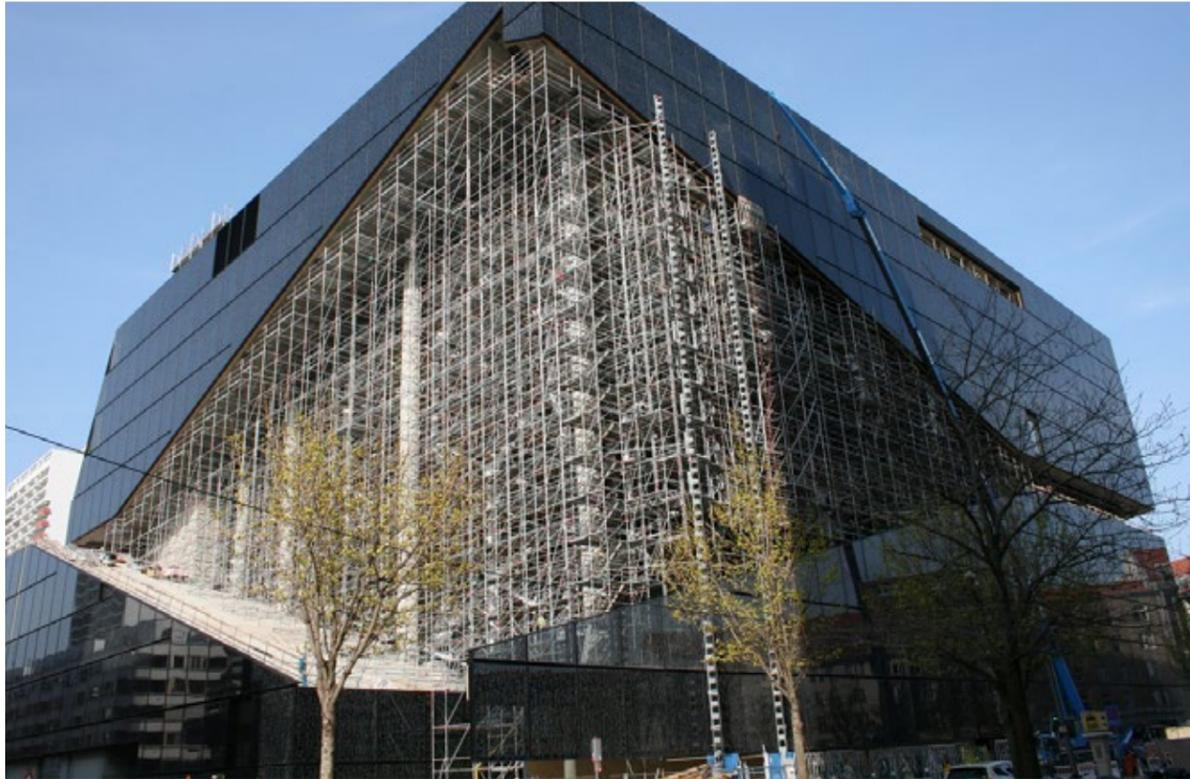
The scaffold initially had a structural function for the atrium, during the final phase of the construction to install the glass panes.
