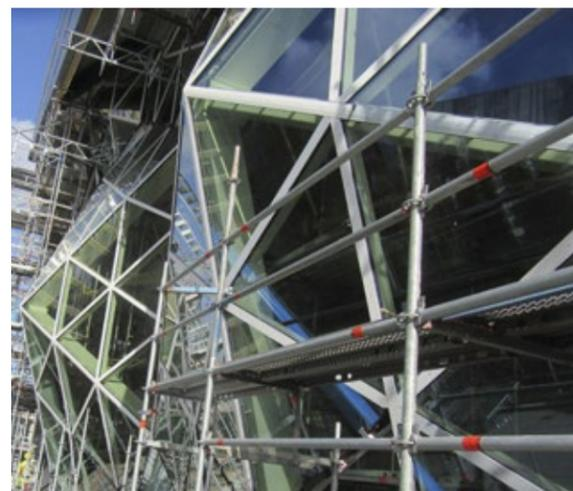
Complex task for the engineering: The glass triangles are three-dimensionally faceted outwards and turned inside out.
