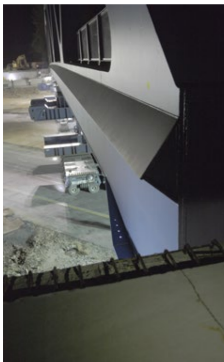
After the bridge was maneuvered next to the supports and stood parallel to their final position, the wheels were turned 90° and the structure moved from the side to its final position.
