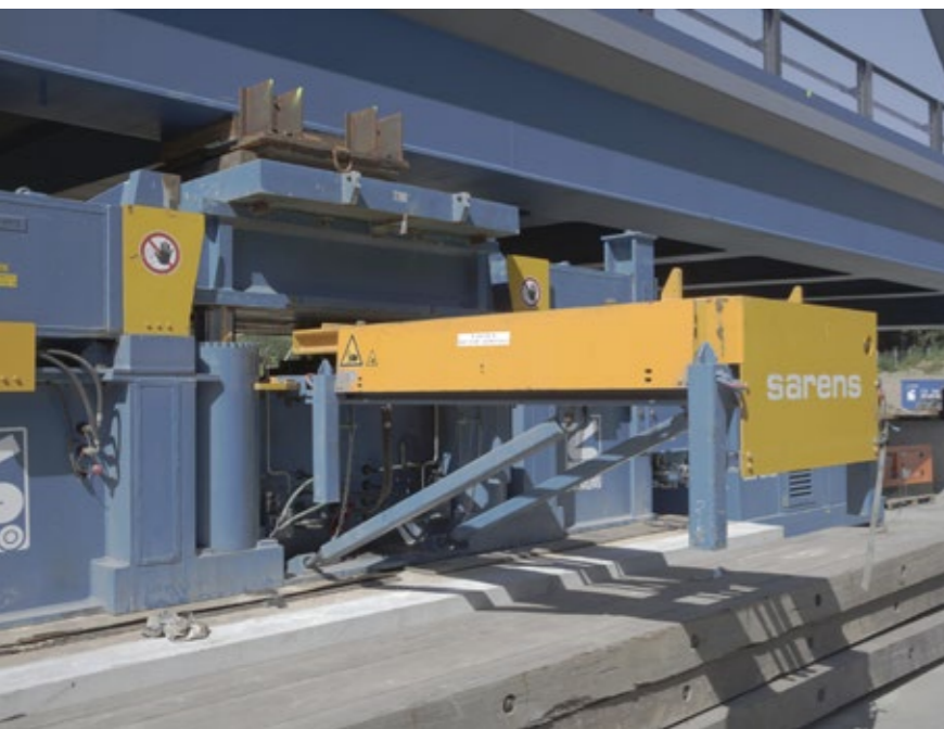
Four such hydraulic lifting presses lifted the bridge.
